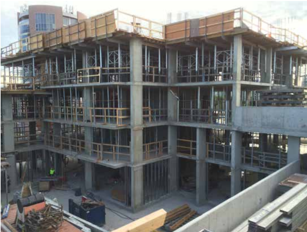
Looking northeast from level 6 southwest
