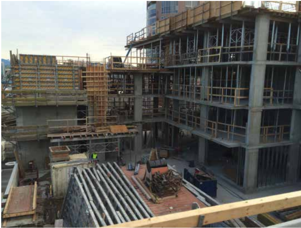
Looking north from level 6 southwest
